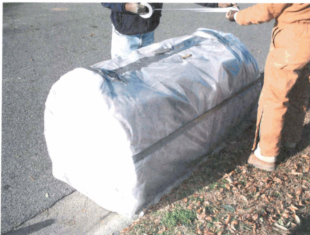
Picture 2: UST 665Camellia being wrapped for disposal.
